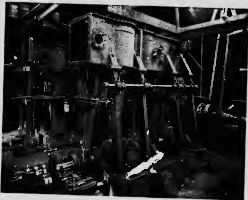
ONE SET OF 1100 H.P. TWIN SCREW TRIPLE EXPANSION MARINE ENGINES IN COURSE OF ERECTION, BAY STREET
