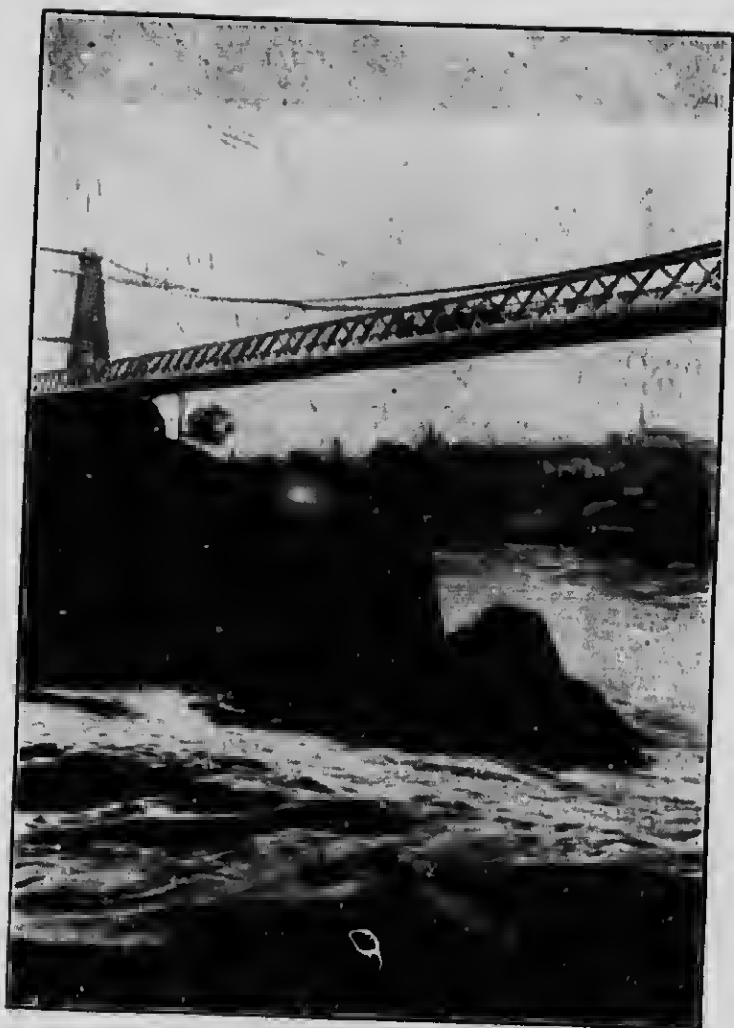
SUSPENSION BRIDGE AT ST. JOHN OVER REVERSING FALLS DARK LINE ON ROCKS SHOWS HEIGHT TO WHICH TIDE RISES WHEN FALL REVERSES.
