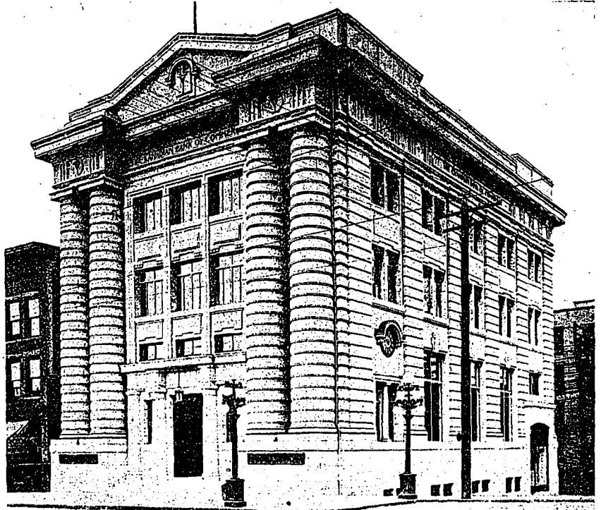
CANADIAN BANK OF COMMERCE (EAST END BRANCH), VANCOUVER, B.C. V. D. HORSBURGH, F.R.I.B.A., ARCHITECT.
