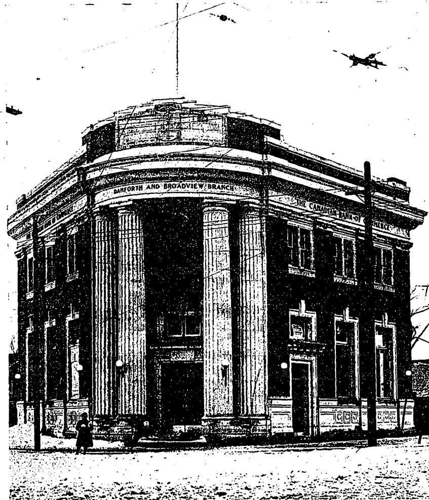
BRANCH OF CANADIAN BANK OF COMMERCE, DANFORTH AND BROADVIEW AVENUES, TORONTO. V. D. HORSBURGH, F.R.I.B.A., ARCHITECT.
