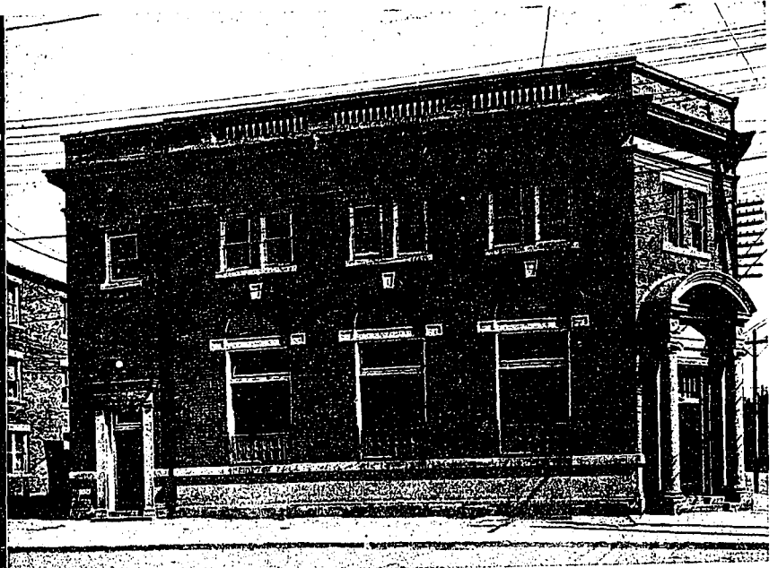
BANK OF TORONTO, ARTHUR STREET AND OSSINGTON AVENUE, TORONTO.
