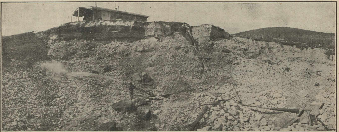
Small Hydraulic Plant on Bonanza Creek.
