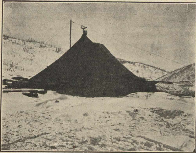
Dump of Pay-dirt Built with Dawson Carrier.
