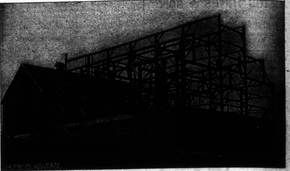
Basement and Frame of Mr. J. A. James' Dairy Stock Barn, Nilestown, Ont. New portion, 72x60 feet. Walls, 12 feet high.
