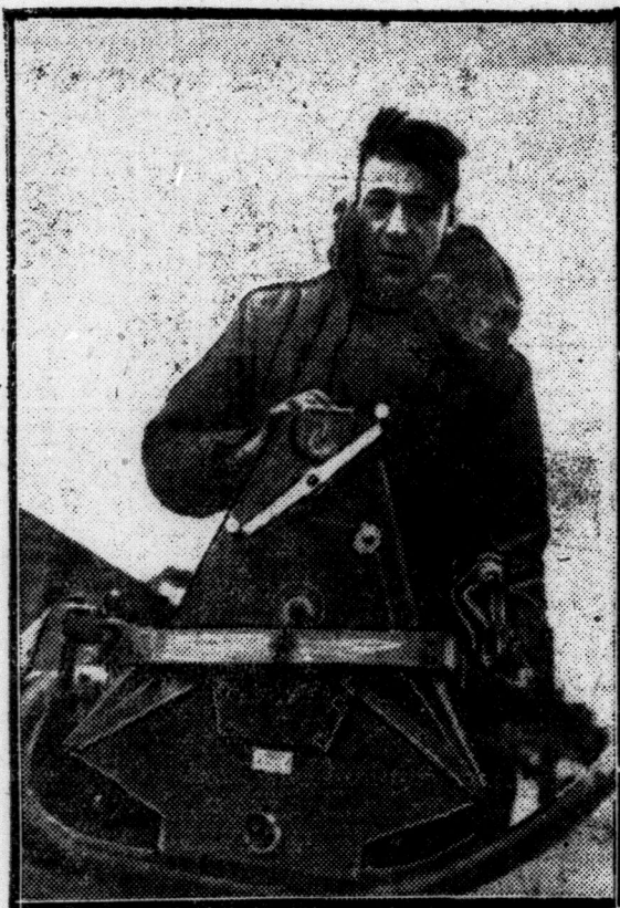
With this new air camera officers in the American army were able to photograph 1,000 square miles in two hours. It is used for map making, uses a roll of film 390 feet long and 6 inches wide and takes in a strip of land ten miles long at one time.
