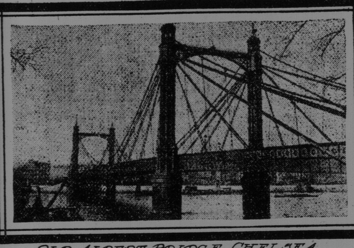
OLD ALBERT BRIDGE CHELSEA
