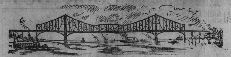
Is Now Under Construction—Will Cross the St. Lawrence River at Quebec—Main Span is 1800 Feet Long and Contains 10,000 Tons of Steel—Cost of the Bridge is \$4,500,000.
