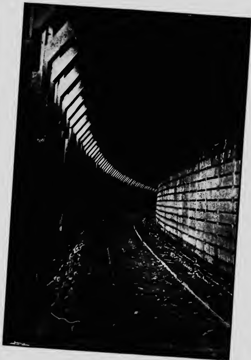
INTERIOR OF A SNOW SHED.
