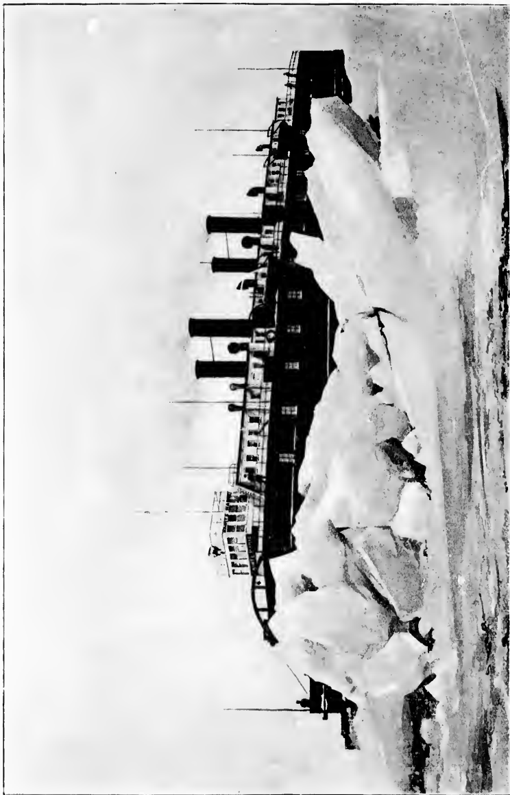
MACKINAW CAR FERRY ICE BREAKER GOING THROUGH THREE FEET OF ICE
