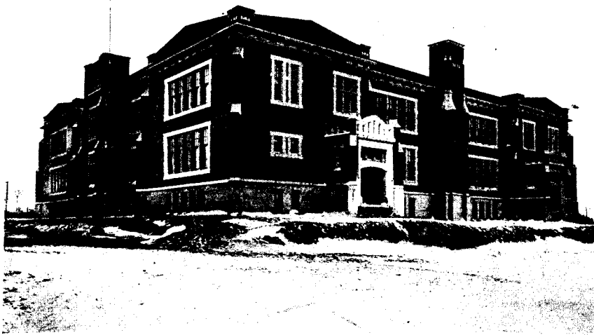
OAKWOOD HIGH SCHOOL, TORONTO. Erected under supervision of C. H. Bishop, Supt. of School Buildings. Brick Contractors, H. Lucas & Son. Contractor for Hollow Tile Fireproofing, Robt. Bennett.
