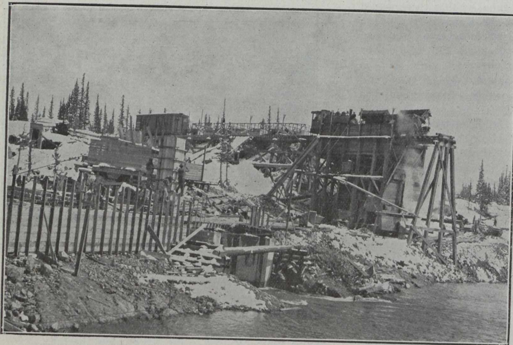
Mixing Plant, as Seen from Southwest Corner of Cofferdam.
