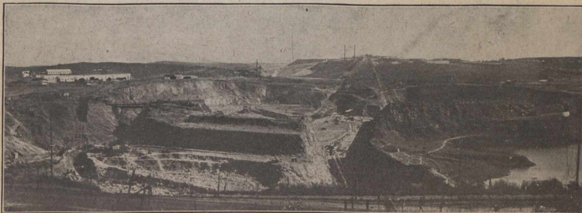
View of Mine from Kopje at back of Native Hospital (looking west). Showing Mine Workings, Nos. 2, 3 and 4 Gears and No. 2 Compound and Fences.
