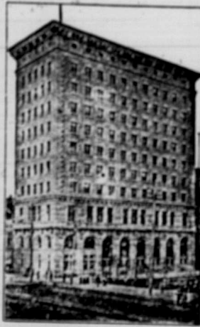
Union Bank Building, Winnipeg
