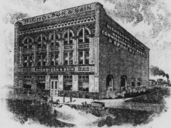
BANNATYNE ST. EAST TRANSFER TRACK.
