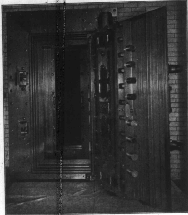
Vault doors in Bank of Montreal and Royal Trust Company, Montreal. Three times larger and heavier than any other in Canada. Doors and Vestibules weigh 60 tons. Total weight of lining and doors 260 tons. Accepted to be the finest piece of vault work in construction and workmanship in the Dominion. — Built by the old established firm of
