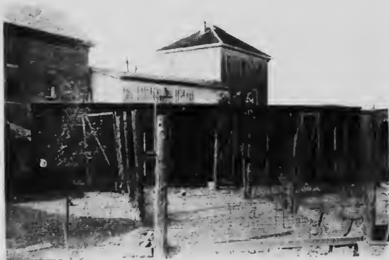
This house is made of building paper laid on poultry netting, without boarding
