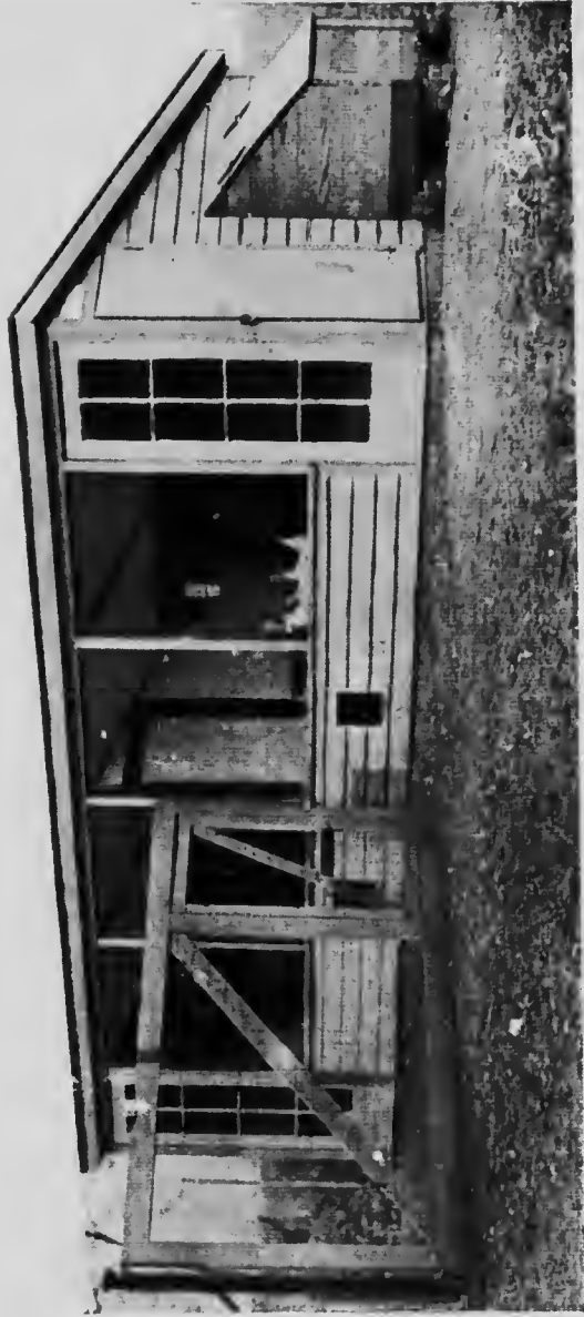
An ideal home poultry plant designed at the Perdue University Experiment Station. The glass window extends almost to the floor and there are muslin curtains for the openings
