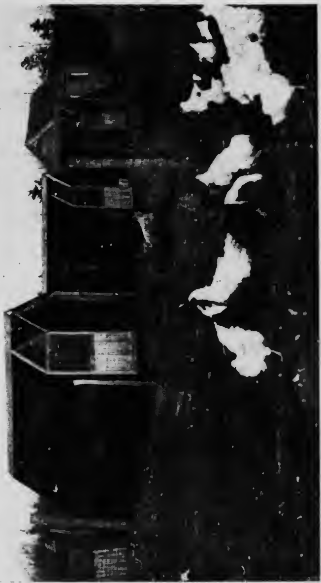
"A" houses of the open-front type are inexpensive and serviceable. Usually they are covered all over with roofing paper
