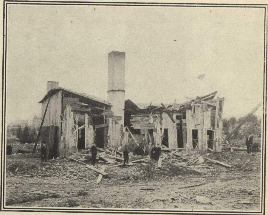
A Cement Mill, over one hundred yards from where the explosion occurred, but which was completely wrecked.
