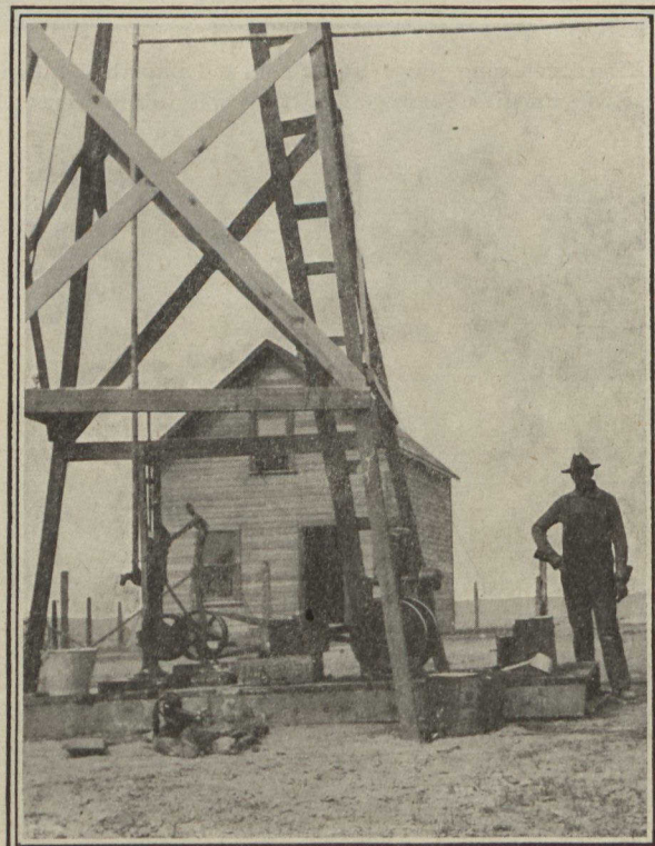
Artesian Well in the Dry Belt, water at 35 feet.
