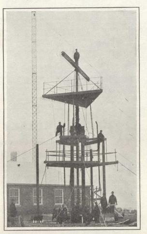
Beginning to Build the Big Steel Tower at Newcastle, Beside Receiving Station. In the distance a 300-foot Wooden Tower Completed.
