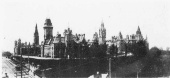
FEDERAL BUILDINGS, OTTAWA.
