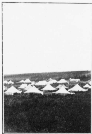
A CHARACTERISTIC RAILWAY CONSTRUCTION CAMP.
