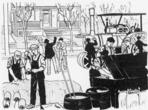
SIX O'CLOCK WITH A ROAD-MAKING GANG.
