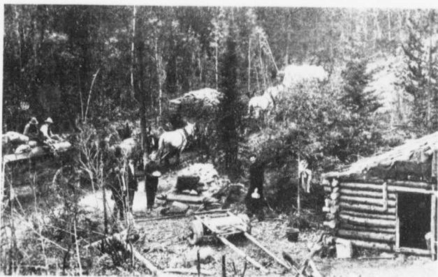
TOTING SUPPLIES FOR CONSTRUCTION IN THE ROCKIES. Stationman's shack, oven and cart.
