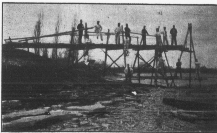
A BRIDGE IN COURSE OF CONSTRUCTION
