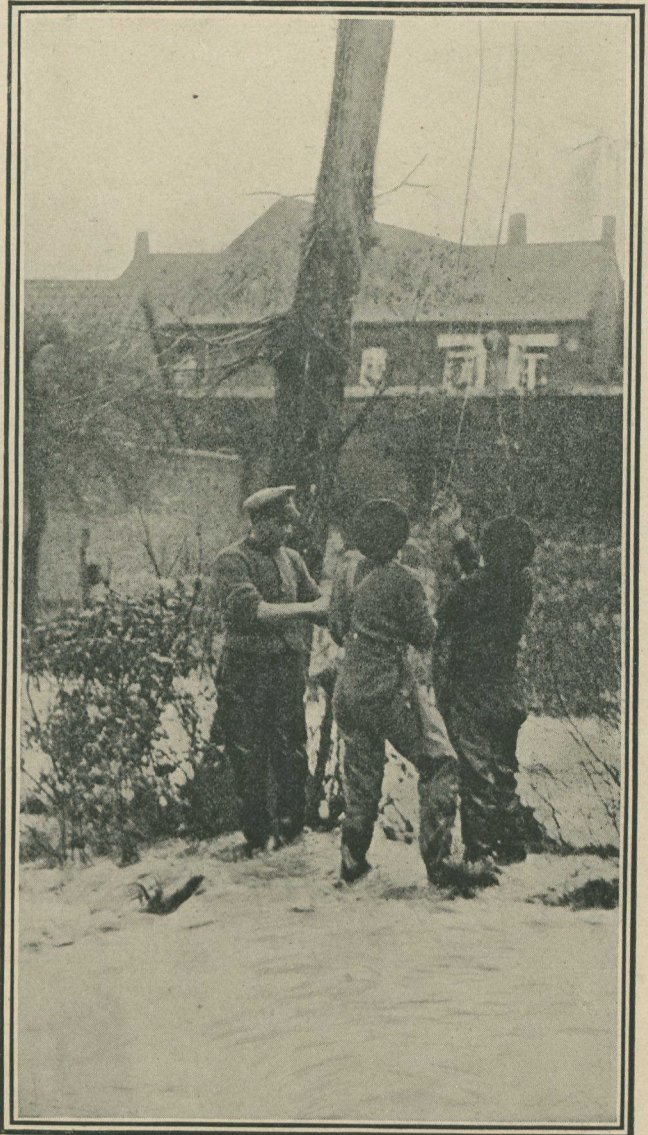
CANADIAN SIGNALLERS REPAIRING TELEPHONE WIRES IN A FLOODED DISTRICT
