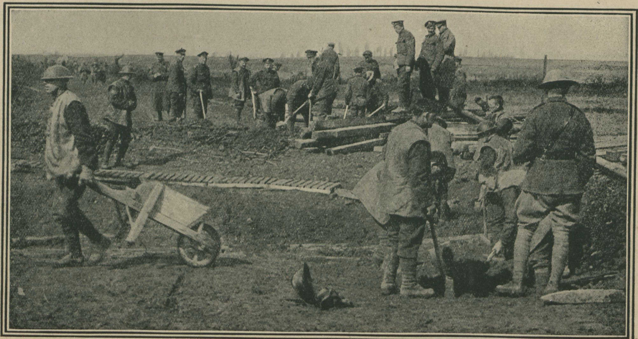
—IN REPAIRING THE DAMAGED ROADS FOLLOWING THE GREAT ADVANCE
