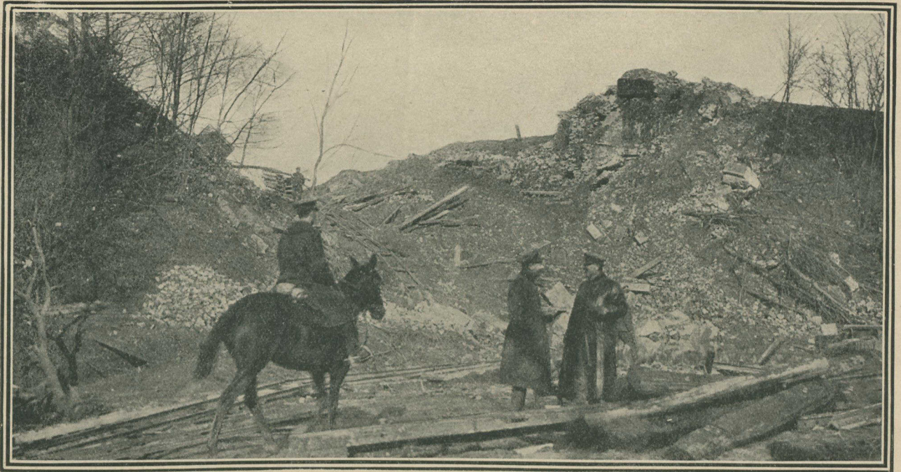
BRIDGE ON THE NESLE-HAM RAILWAY BLOWN UP BY THE RETREATING HUNS
