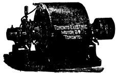
Our new four-pole Motors, highest efficiency and all latest improvements; built in sizes 10 to 50 h. p. Our Bipolar Motors from 3 to 20 h. p. are not equalled Electric Elevators, freight or passenger, contracted for—power or direct connection.
