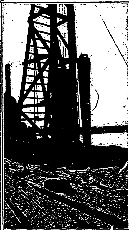
FIG. 4—TEST PILE PARTIALLY DRIVEN SHOWING WOODEN PILE ALONGSIDE.
