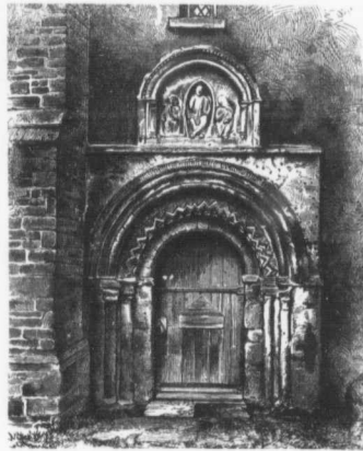
OLD NORMAN TOWER, ELSTOW CHURCH.
