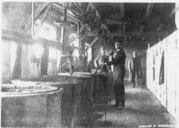
Rendering Room where the Fish Waste was Treated to Separate the Valuable Oil Content, Port Dover, Ont.
