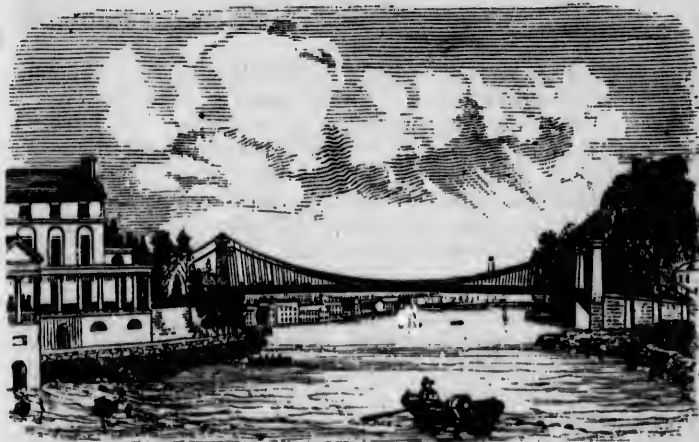
Suspension Bridge over the Schuylkill River, with part of Fairmount.
