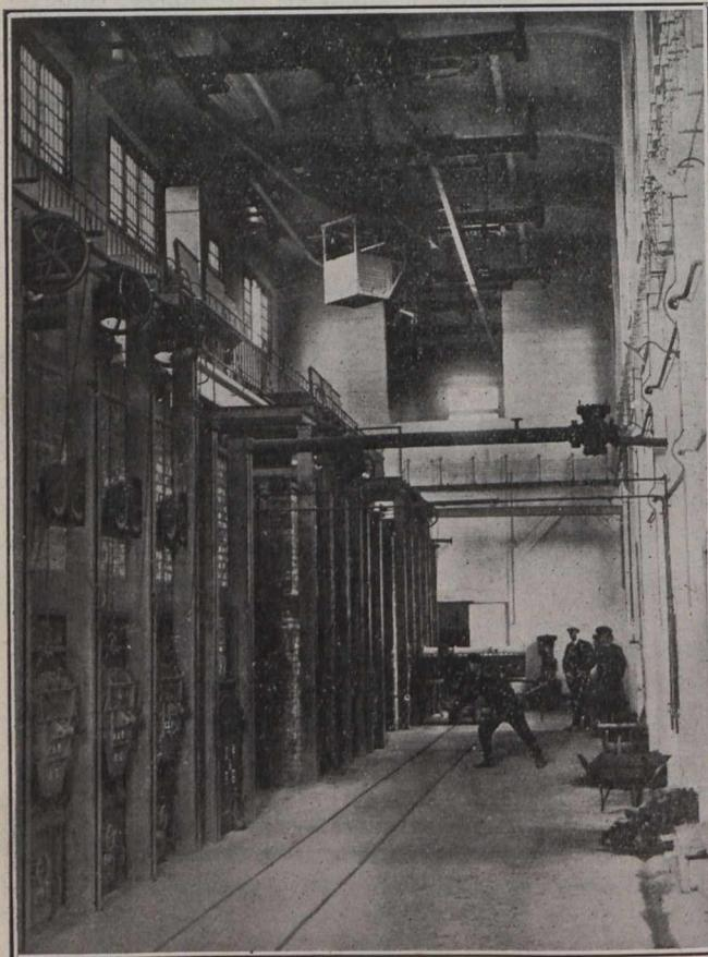
Fig. 2.—View of Clinkering Floor Showing Method of Withdrawing Clinker.
