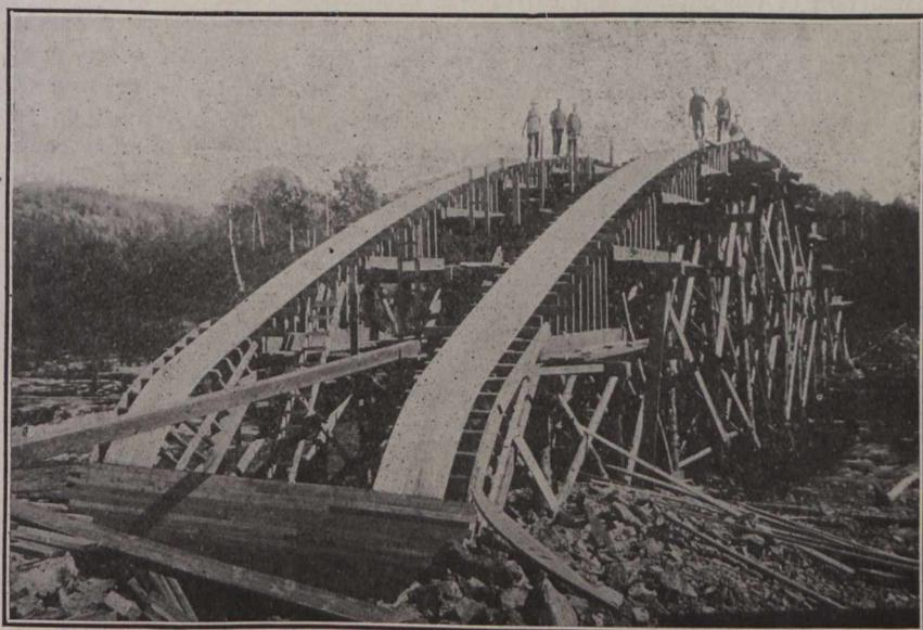
View Showing Forms for Ribs Ready to Put Forms for Slides in Place.
