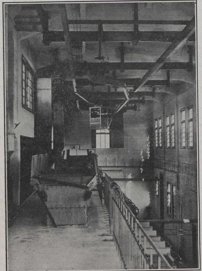
Fig. 3.—Charging Floor Showing Top of Containers from Which Refuse is Charged.
