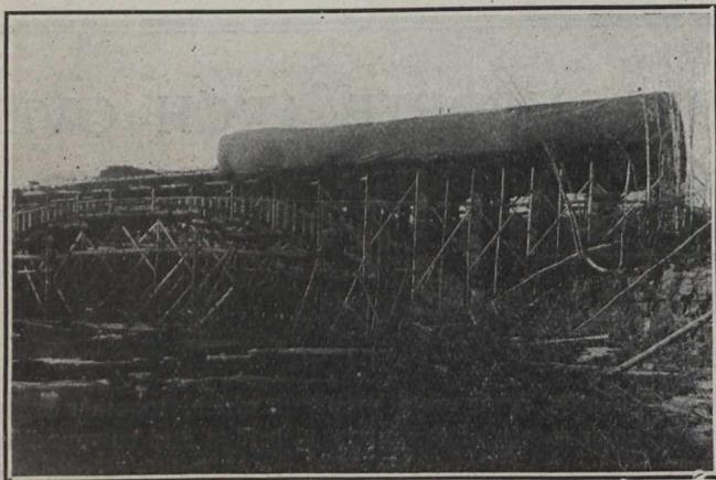
View Showing Covering for Finishing Walks and Surfaces During Cold Weather.
