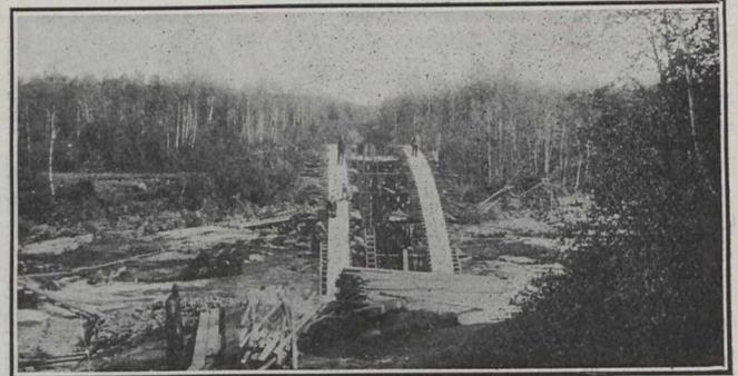
View Showing Formwork of Ribs and General Surroundings.
