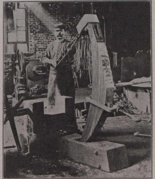
Powerful Screw Operated Clamp for Tightening up Spring Bands.
