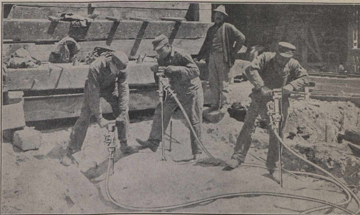
"Three 'Busy Bees' at work on the New York Subway Excavation."
