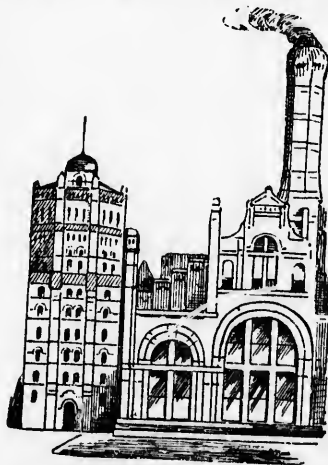
CORLISS ENGINEHOUSE AND WATER TOWER.
