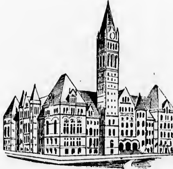
TORONTO MUNICIPAL BUILDINGS.
