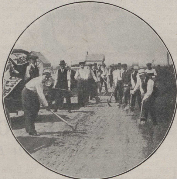
How the Moncton Business Men Showed Their Determination to Help Along the "Good Roads" Movement.
