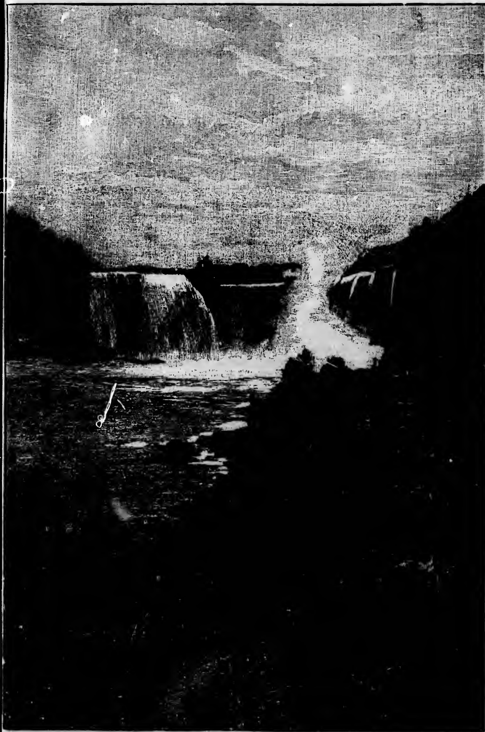
HORSESHOE FALL FROM THE FERRY ROAD.
