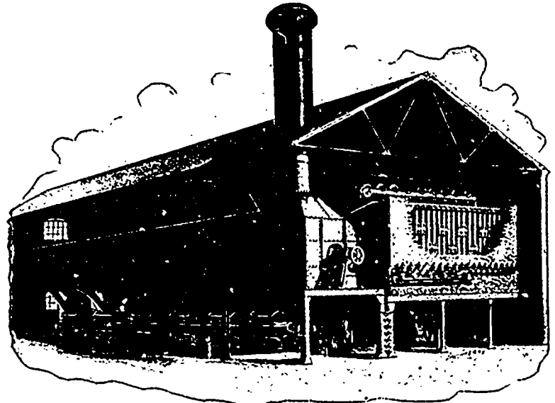
A Central Power Station, with induced draft, economizers, etc.
