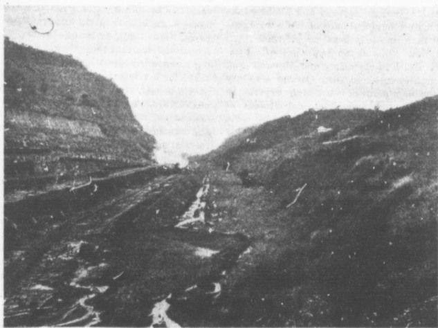
The famous Culebra Cut, Panama Canal, showing the excavation already accomplished.
