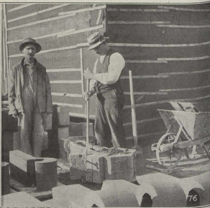
Fig. 10.—Tamping Concrete in the Forms.
