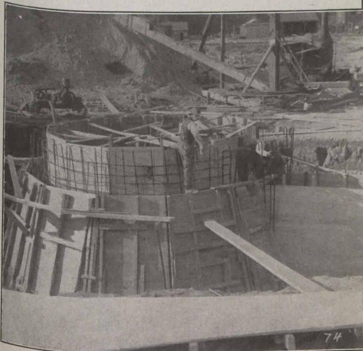
Fig. 6.—Forms for Foundations.
