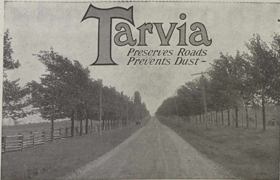
Kennedy Road, Scarboro Township, York County, Ontario. Tarvia filled macadam.
