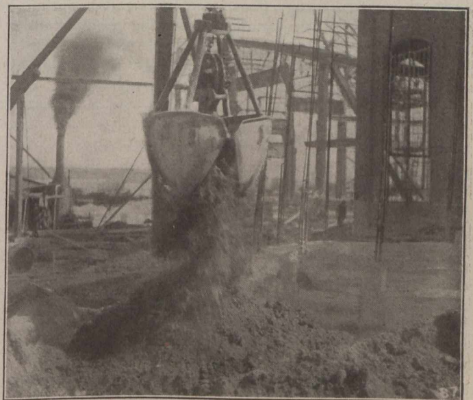
Fig. 8.—Backfilling Around Foundations with Hayward Bucket.
