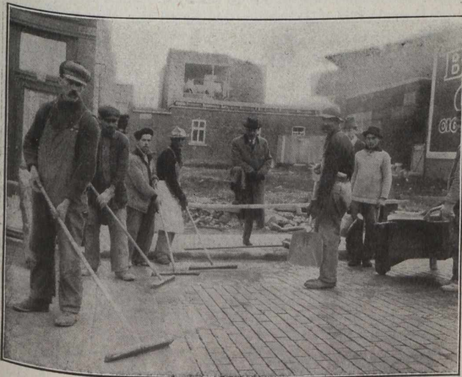
Fig. 2.—Applying Cement Grout Filler at Outremont, P.Q.
