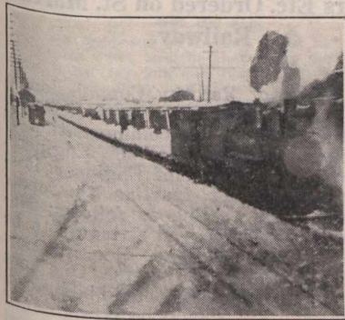
Fig. 3. Removing Snow Between Tracks.
