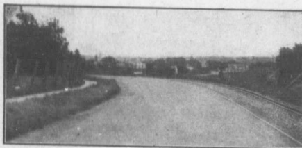
This is Merriton Road in St. Catharines, an important thoroughfare running through the manufacturing district between St. Catharines and Merriton, resurfaced with "Tarvia-X," and with "Tarvia-B" seal coat in 1917.
