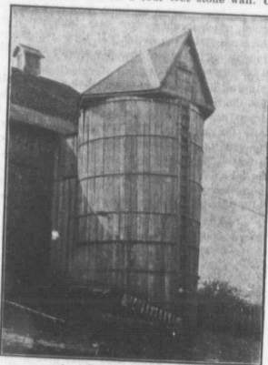
1—A Representative Stave Silo
