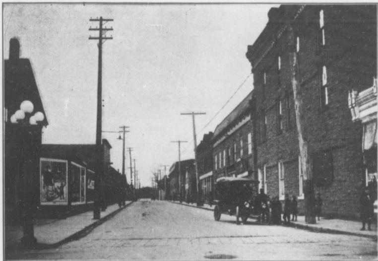
PERTH STREET LOOKING NORTH FROM KING STREET.
