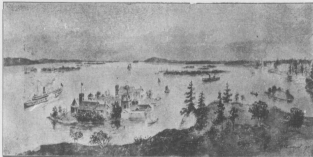
BROCKVILLE'S ISLAND PARK.
