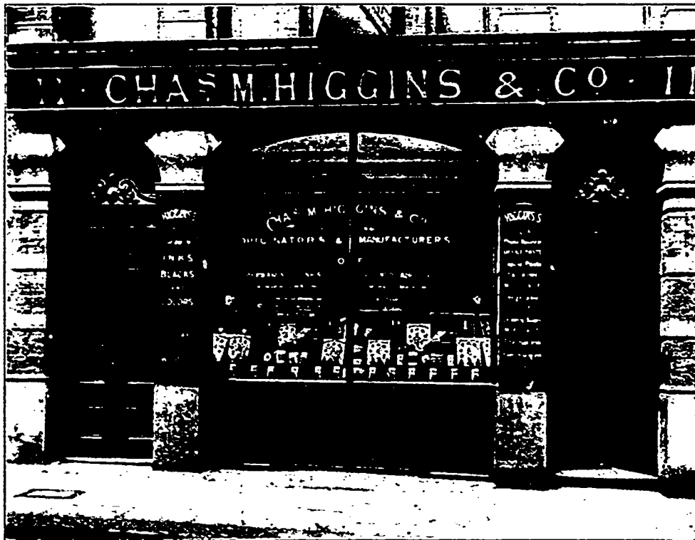
LONDON BRANCH, 11 FARRINGDON AVENUE, LONDON, E.C.—(Store and Basement, each 25 x 75)
