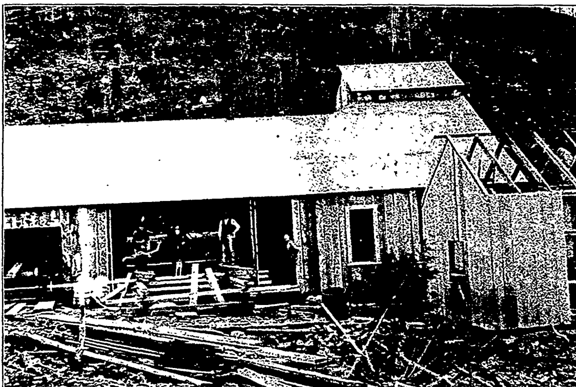
Engine and Shaft House, Josie Mine, B. C.
