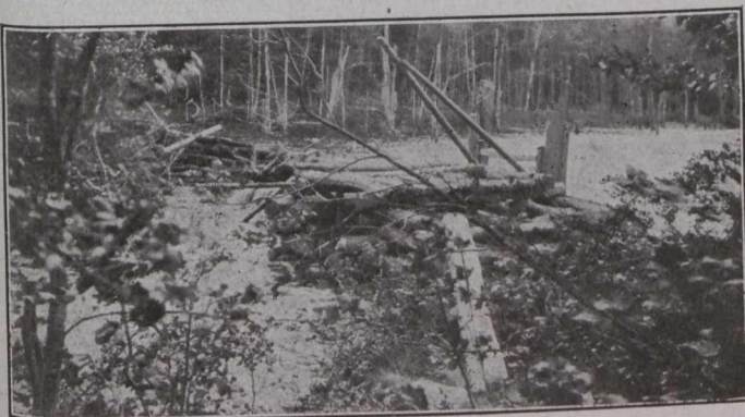
Sackville River—A Typical Log-driving Dam.
