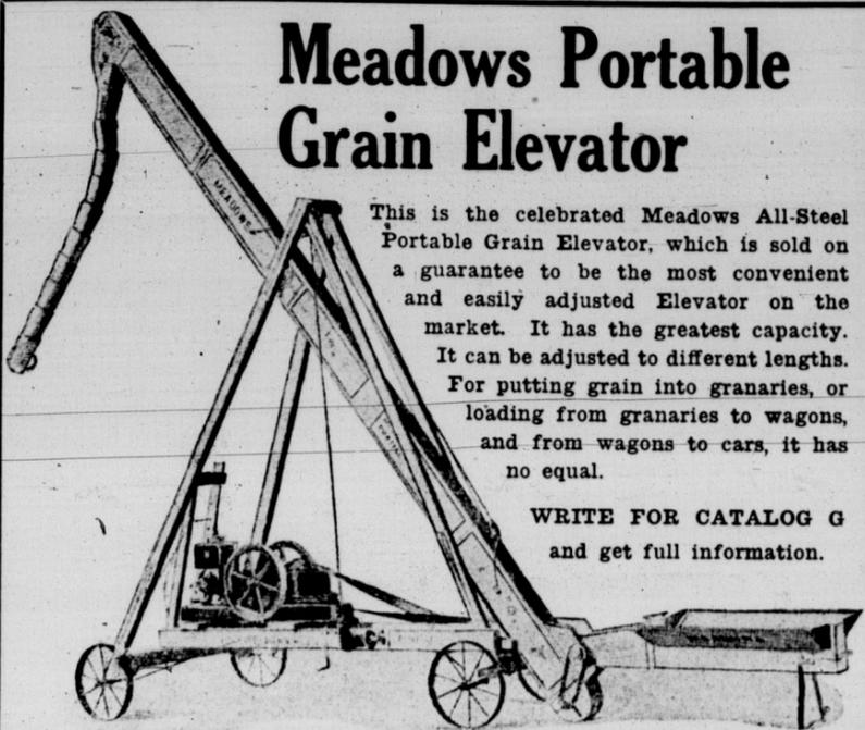
This is the celebrated Meadows All-Steel Portable Grain Elevator, which is sold on a guarantee to be the most convenient and easily adjusted Elevator on the market. It has the greatest capacity. It can be adjusted to different lengths. For putting grain into granaries, or loading from granaries to wagons, and from wagons to cars, it has no equal.
