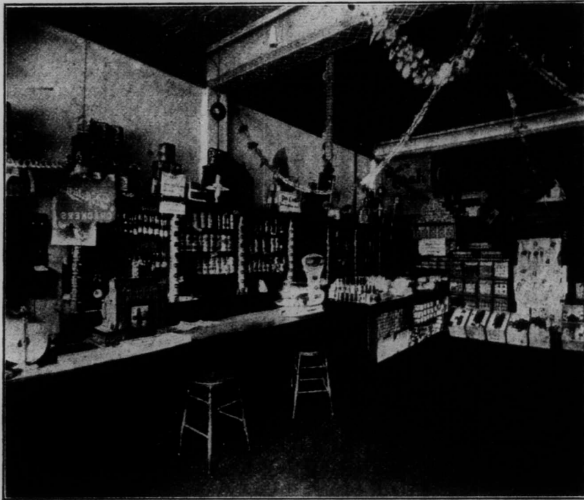
ONE OF THE STORES BURNED AT FERNIE, B.C.
