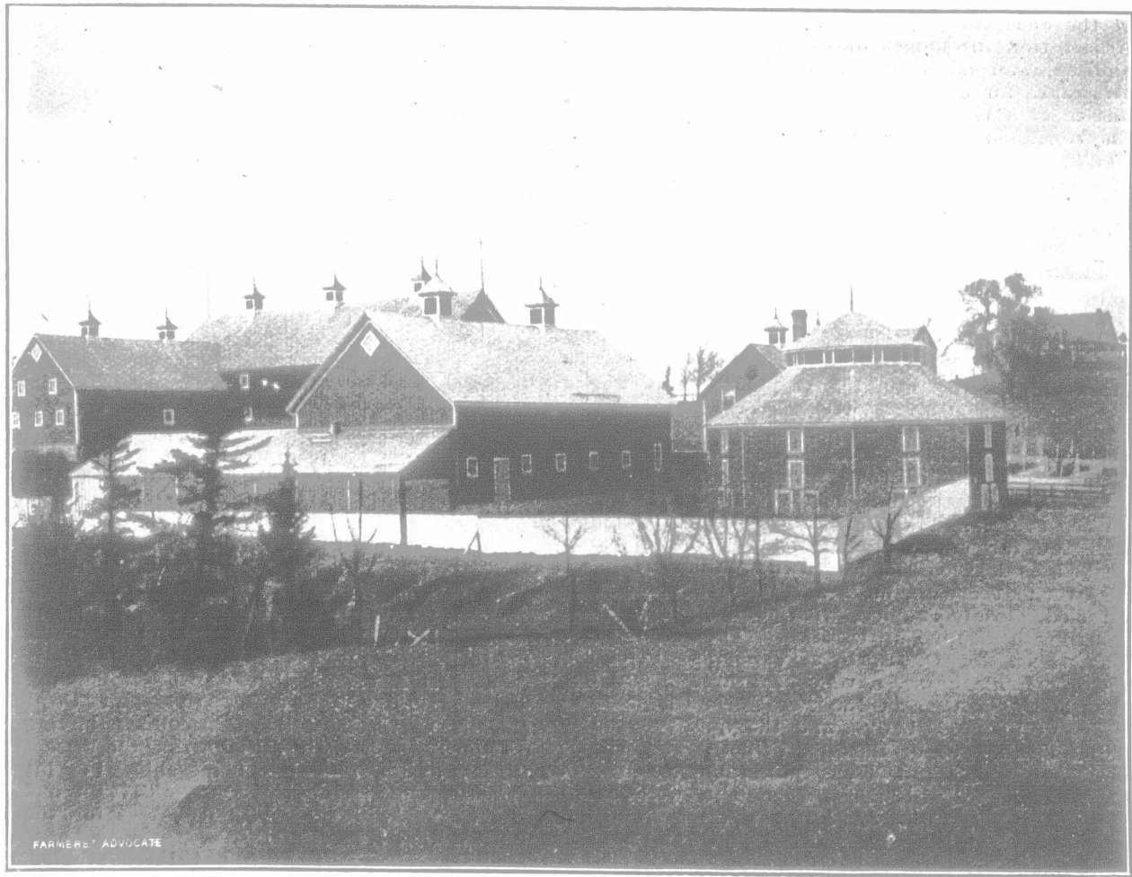
BUILDINGS ON THE PROVINCIAL GOVERNMENT FARM, TRURO, N. S.
