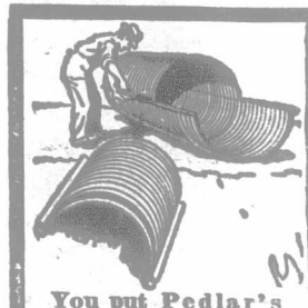
You put Pedlar's Perfect Corrugated Culvert up like this—right at the job
