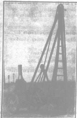
FOR Drilling water wells, or testing mineral land. Run by steam, gasoline or traction engine. Drills wells from two to sixteen inches in diameter.
