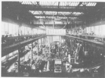
Interior, Main Building, Algoma Iron Works, Limited.
