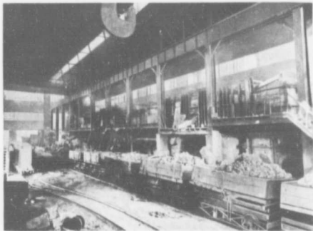
Interior Open Hearth Plant.
