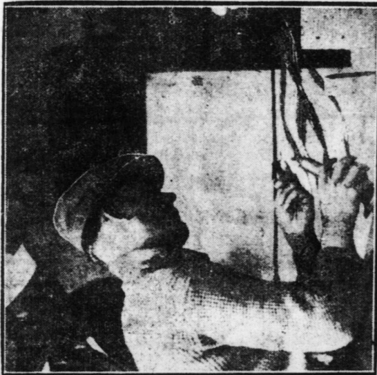
The first splice in the new cable which is being laid between Alaska and Seattle, a distance of 955 miles.
